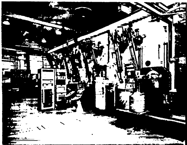
Fig. 401-4. View of Operating Area at the DP-West Facility.
